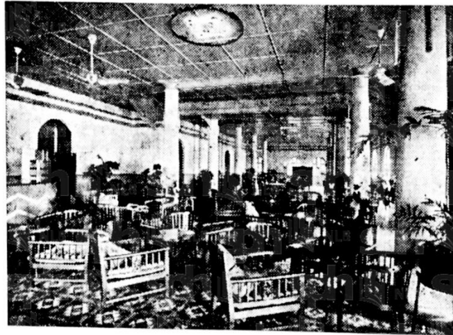
The cocktail bar, lounge and grill room at the Selangor Club Chambers .
